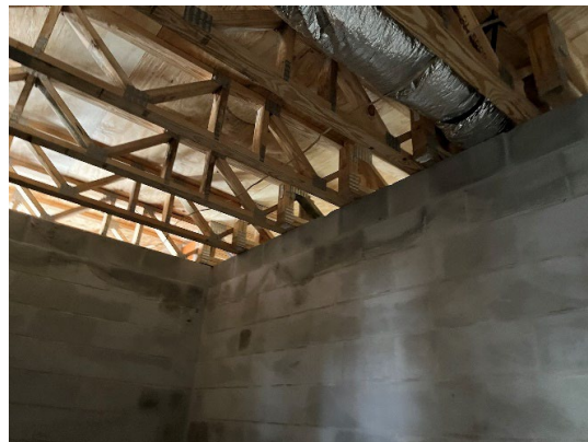
Floor Truss bearing on CMU wall
