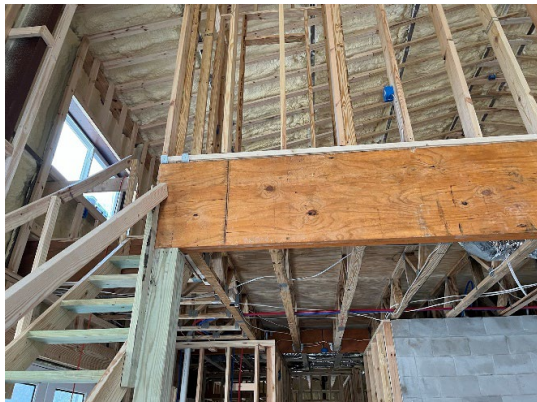
Insufficient Beam Column and Footing (C2)
