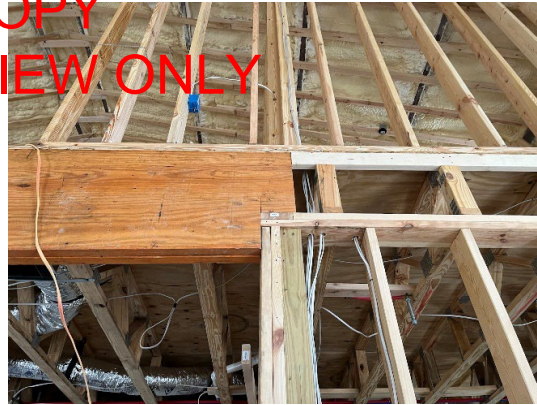
Insufficient Beam Column and Footing (C1)
