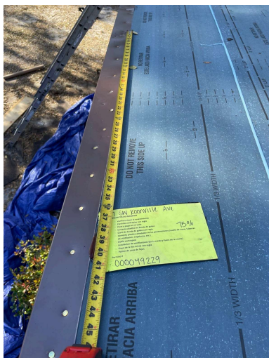
Bannister 7542 Flat Roof 337 SW Koonville Ave • Lake City, FL 32024 Tue, Feb 27 03:42 pm by Jody Simmons
