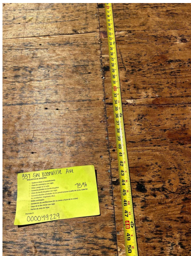
Bannister 7542 Flat Roof 337 SW Koonville Ave • Lake City, FL 32024 Tue, Feb 27 12:30 pm by Jody Simmons
